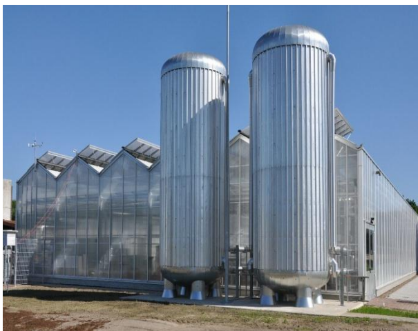
Fig. 1: ZINEG greenhouse with warm and cold water storage, finished May 2010
